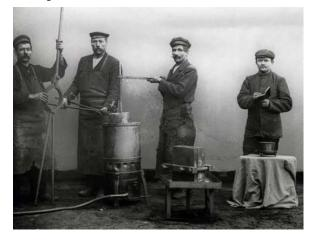
Figure 2: Wilhelm Rohn introduced vacuum metallurgy at Heraeus in 1912. In specially developed electric resistance furnaces, refractory base metals were melted under vacuum to produce entirely new alloys such as chromium-nickel alloys as an alternative to platinum wires in thermocouples, or nickel-iron alloys for components in transmitter and receiver systems in communications engineering. From the 1920s onwards, Heraeus used induction furnaces to produce base metal alloys by the barrel.
